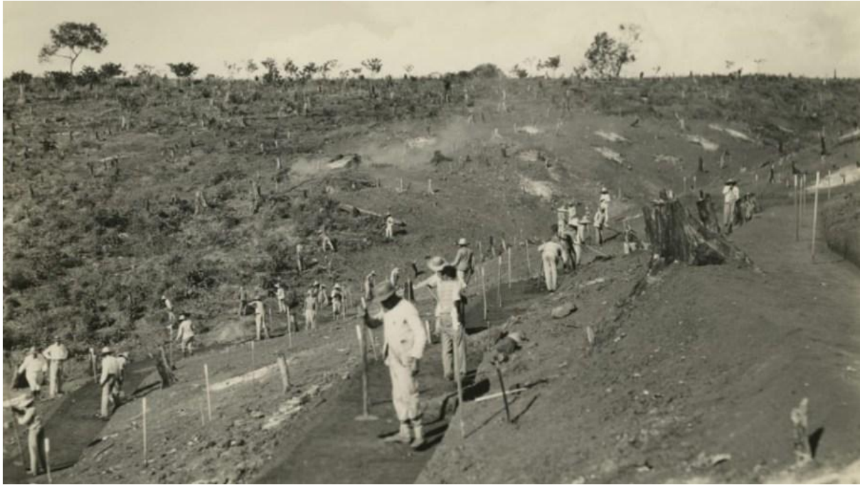
A 1931 photo of workers terracing the land in Fordlandia, Brazil. (Henry Ford Museum)
