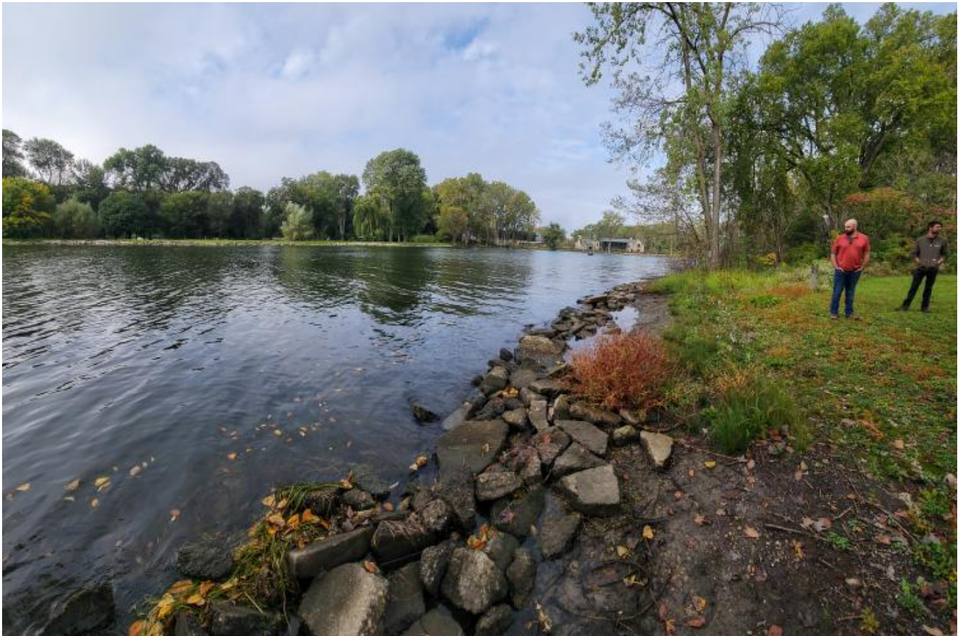
Shoreline hardening at Ford House prior to construction. Credit: NOAA Fisheries/Terry Heatlie
