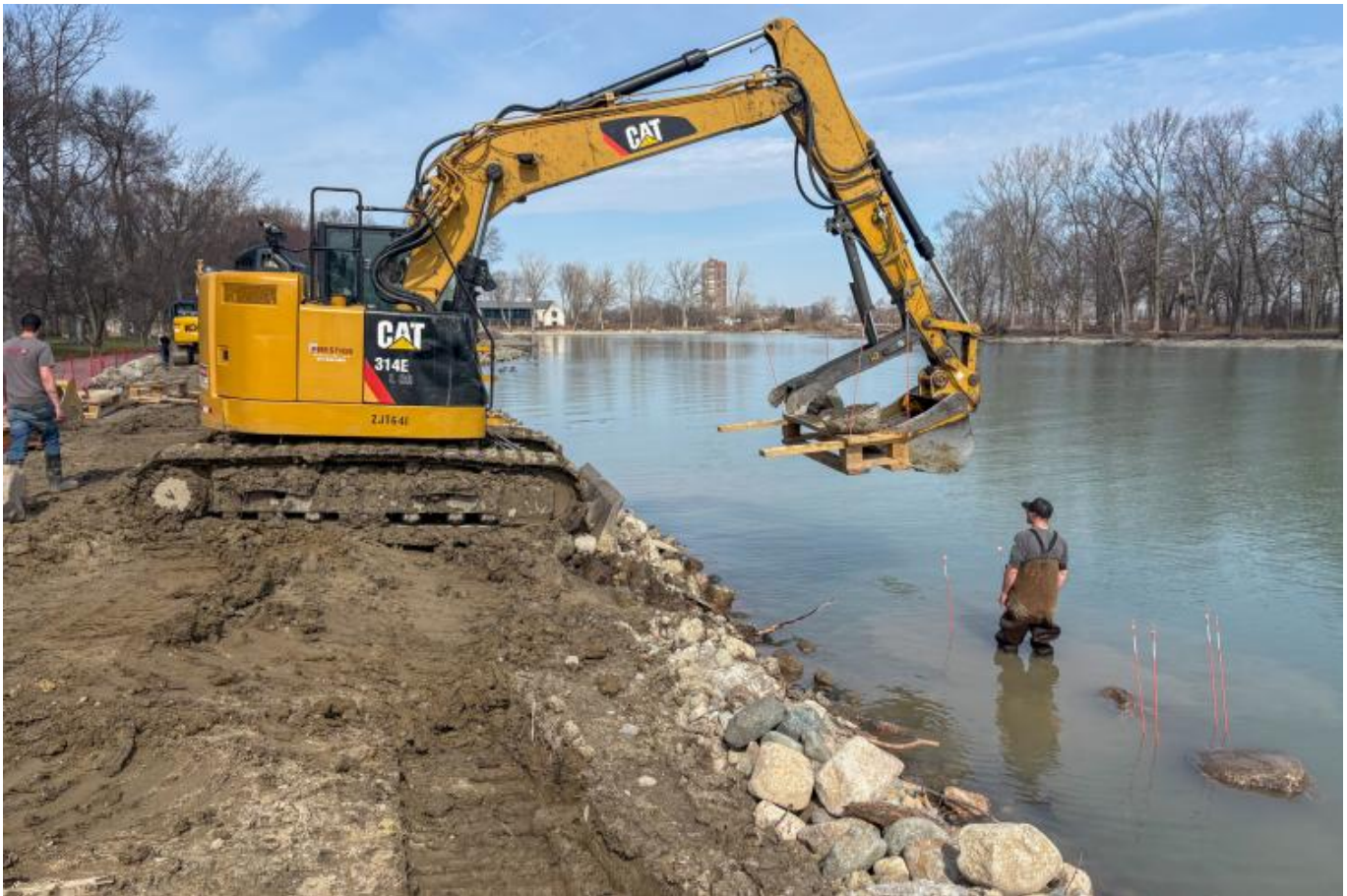
Excavator installing a fish lunker on Ford Cove. Credit: Ford House
