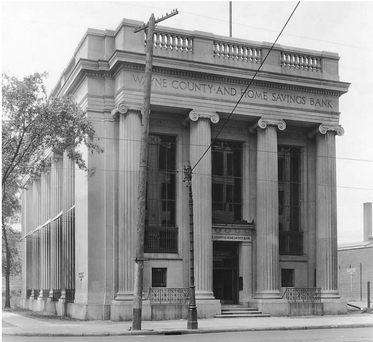
The Wayne County and Home Savings Bank designed in 1915 by Albert Kahn's firm is typical of the Classical style of banks of the period. (Indiana Limestone Photograph Collection)
