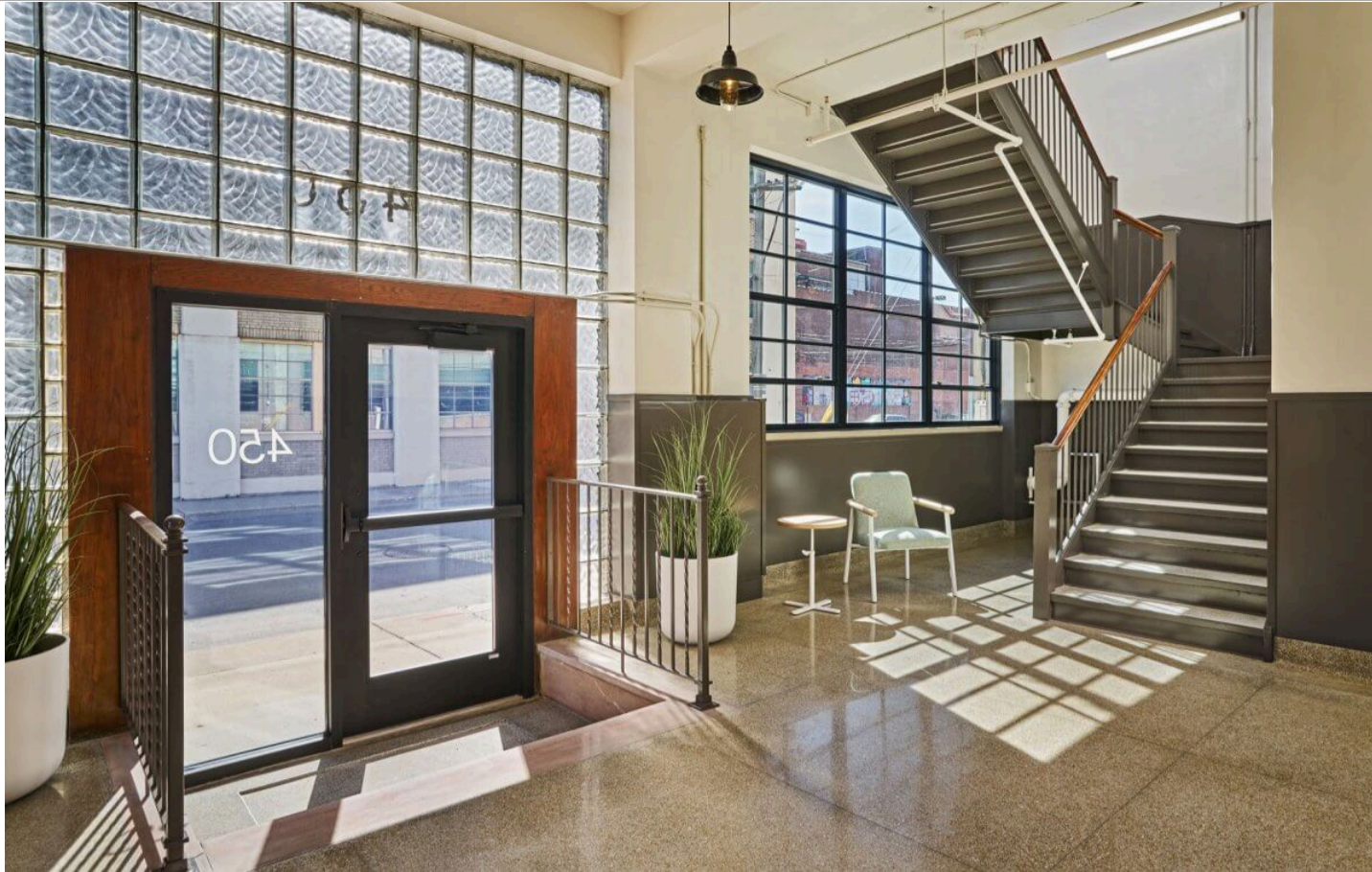
Original glass block encasing an entryway was preserved. (John D'Angelo)
