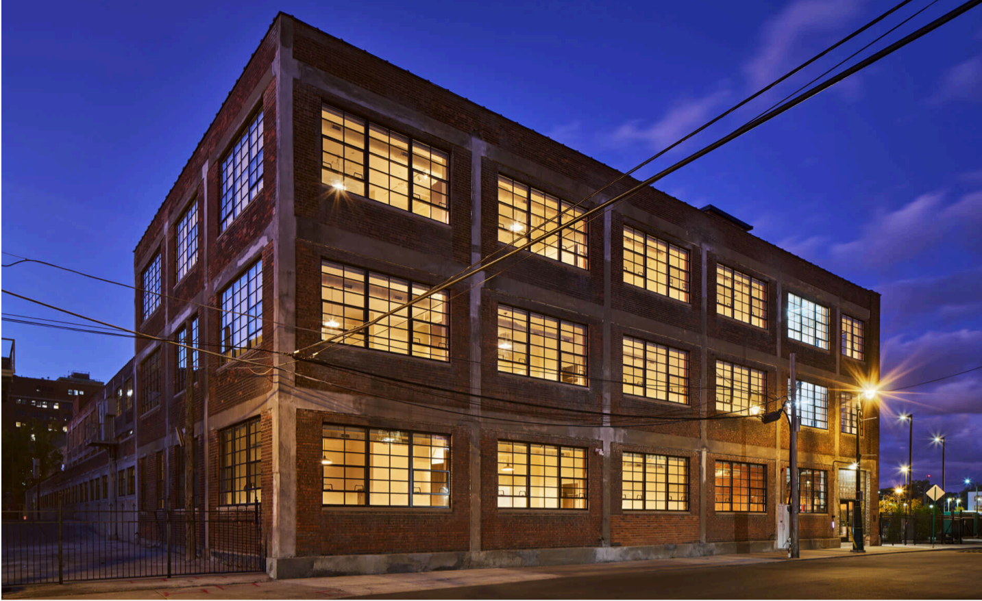
The former Cadillac assembly plant was built in 1905. (John D'Angelo)
