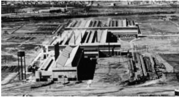
Section of the River Rouge Plant with sawtooth roof
