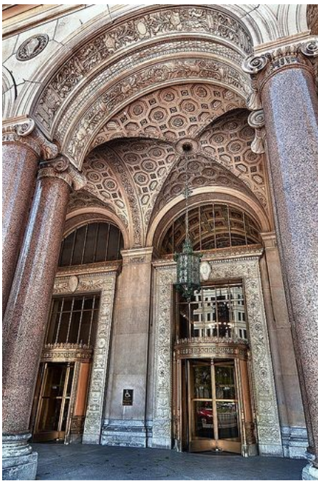
GM Building entrance (Photo by Michael G. Smith via Flickr)
