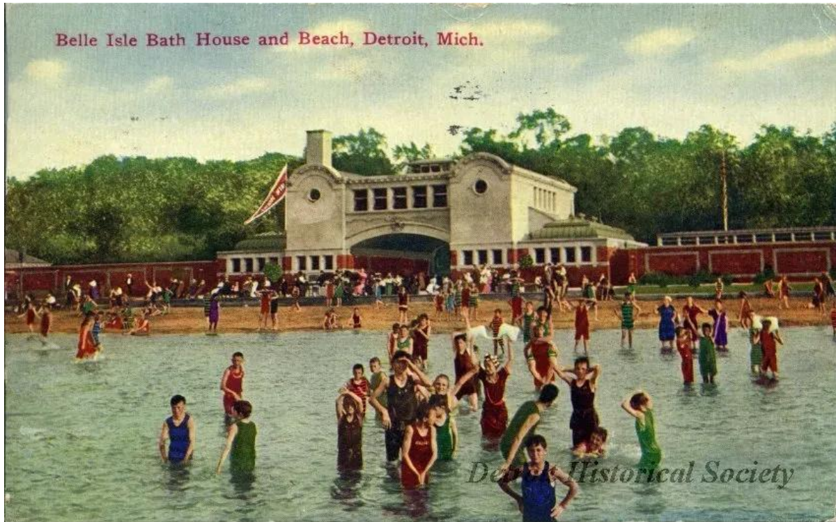
c. 1910 color postcard depicting the Bath House on Belle Isle, with swimmers and the Detroit River in the foreground. Printed on verso: The New Bath House on Belle Isle is the most beautiful building of its kind in the country. It was erected in 1908 at a cost of about $50,000 and has accommodations for 1,300 people. A minimum charge is made and patrons are supplied with suits and towels. The scene here depicted is a common occurrence on a warm summer's day. Detroit Historical Society collection
